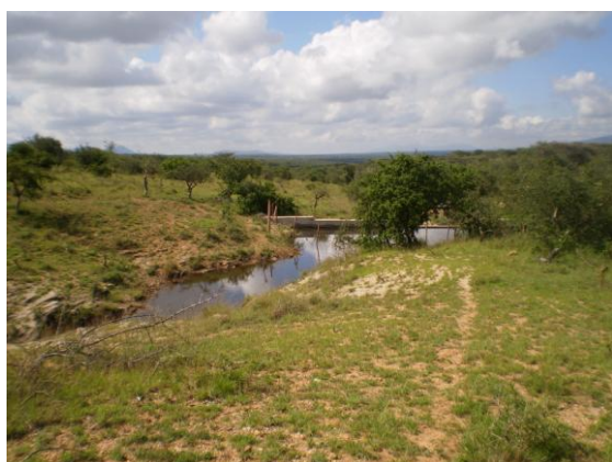
Small stormwater capturing weir on the edge of Kajiado town
